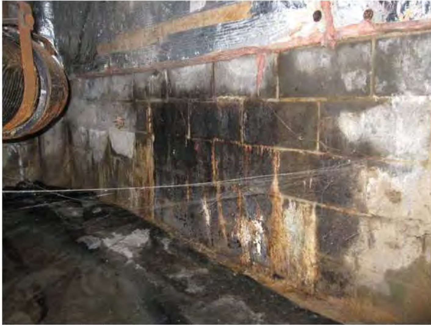
Figure 6 in the NW corner solution deposits have accumulated where rainwater runs down walls from above.
